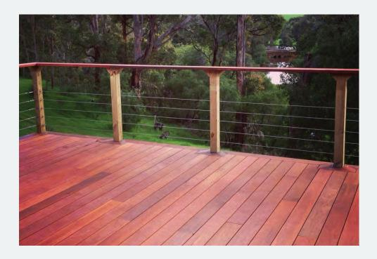
Mortlock Timber uses Cutek CD50 oil when preoiling. Whilst there are other products you can use, below is a recommendation for maintaining your timber decking using Cutek CD50. First coat of Cutek CD50 Clear should be applied to all surfaces of the timber prior to delivery by Mortlock Timber, with a second coat of Cutek CD50 applied once installation is complete.
